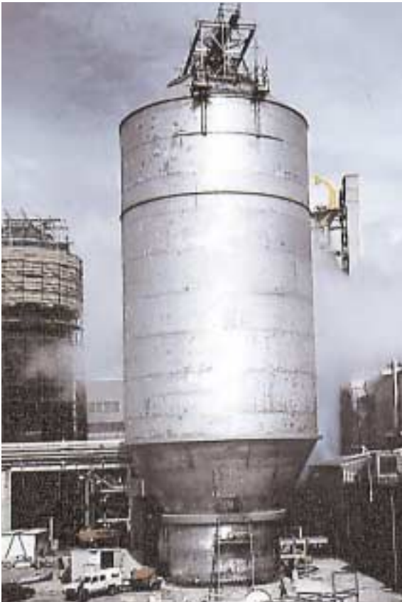
2304 Storage Tank for Forest Products, New Zealand (Source: Usinor Industeel)
